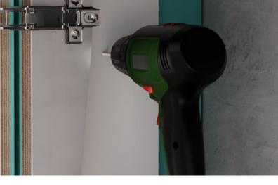
When a return is used to connect a Hygipod to another, drill a pilot hole through one to ensure a tight connection between units.
