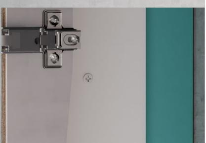
Ensuring the Hygipod is aligned correctly, secure in place using a 4 x 30 mm screw. Secure at the top, middle and bottom.
